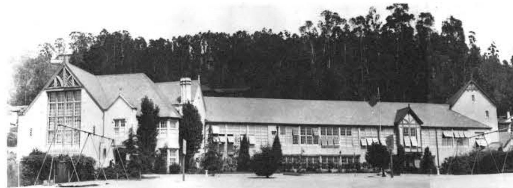
West Elgin - Hillside School Berkeley 4-21-33 West.
