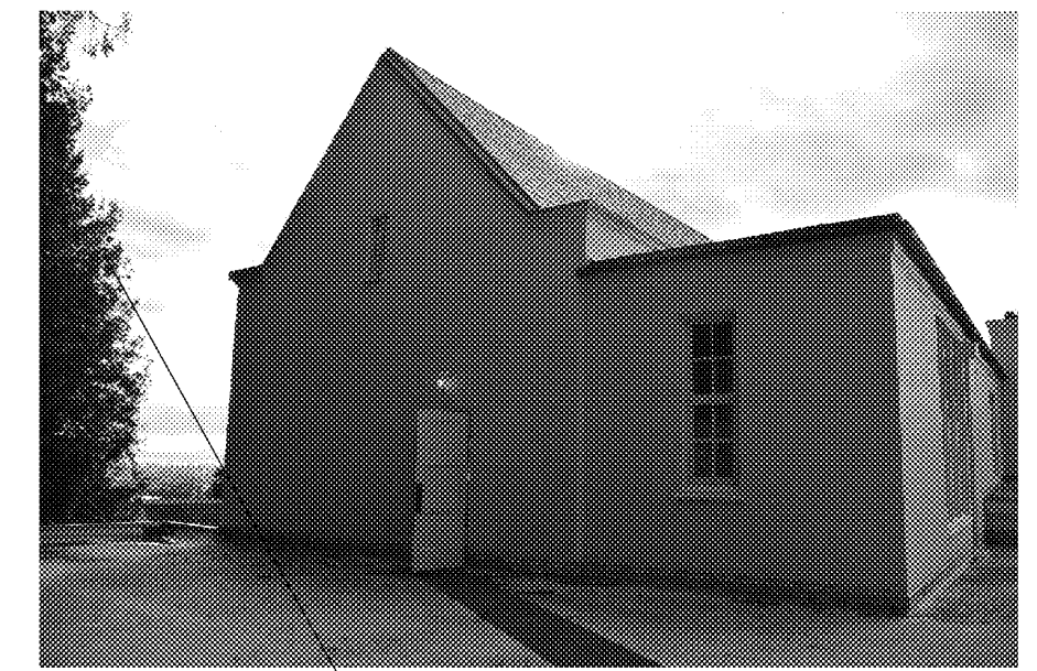
EAST ELEVATION PHOTO
