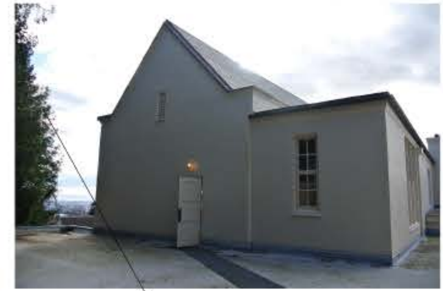
EAST ELEVATION PHOTO
