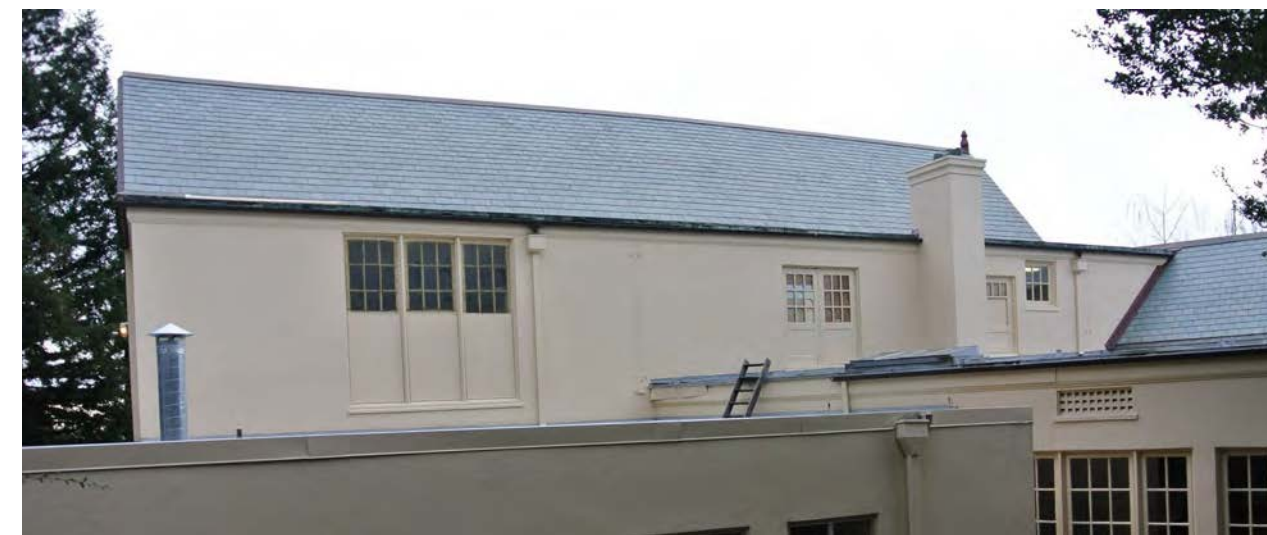
NORTH ELEVATION PHOTO
