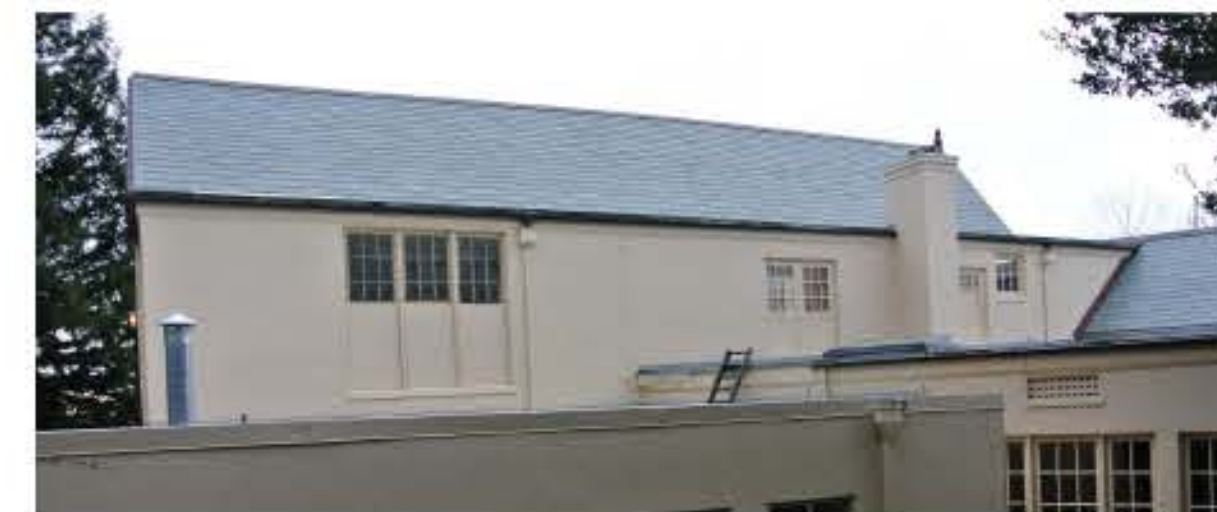
NORTH ELEVATION PHOTO
