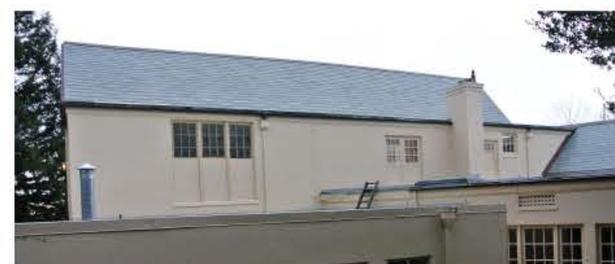
NORTH ELEVATION PHOTO
