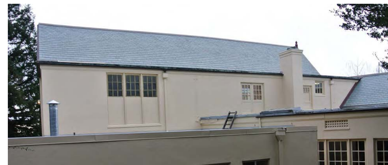
NORTH ELEVATION PHOTO
