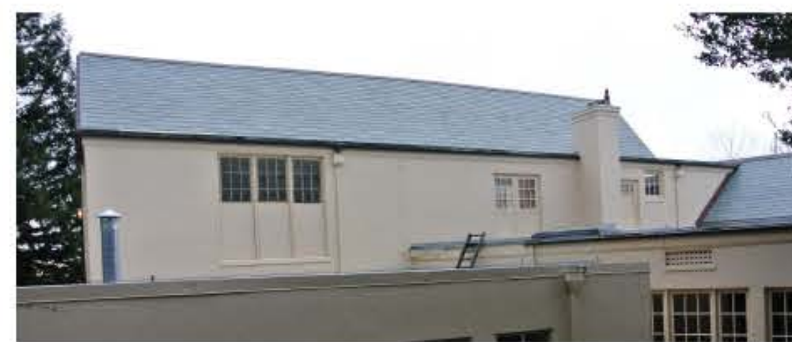
NORTH ELEVATION PHOTO
