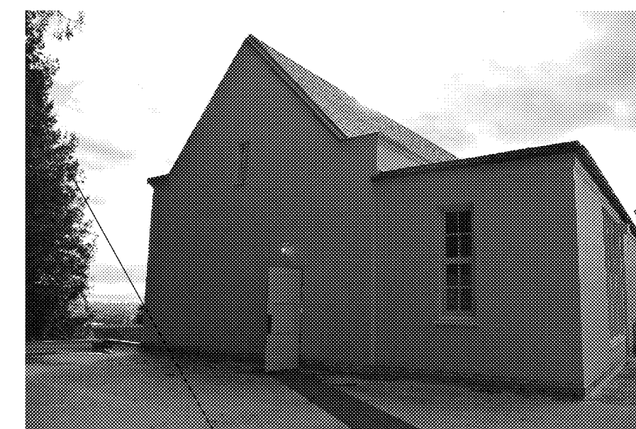
EAST ELEVATION PHOTO
