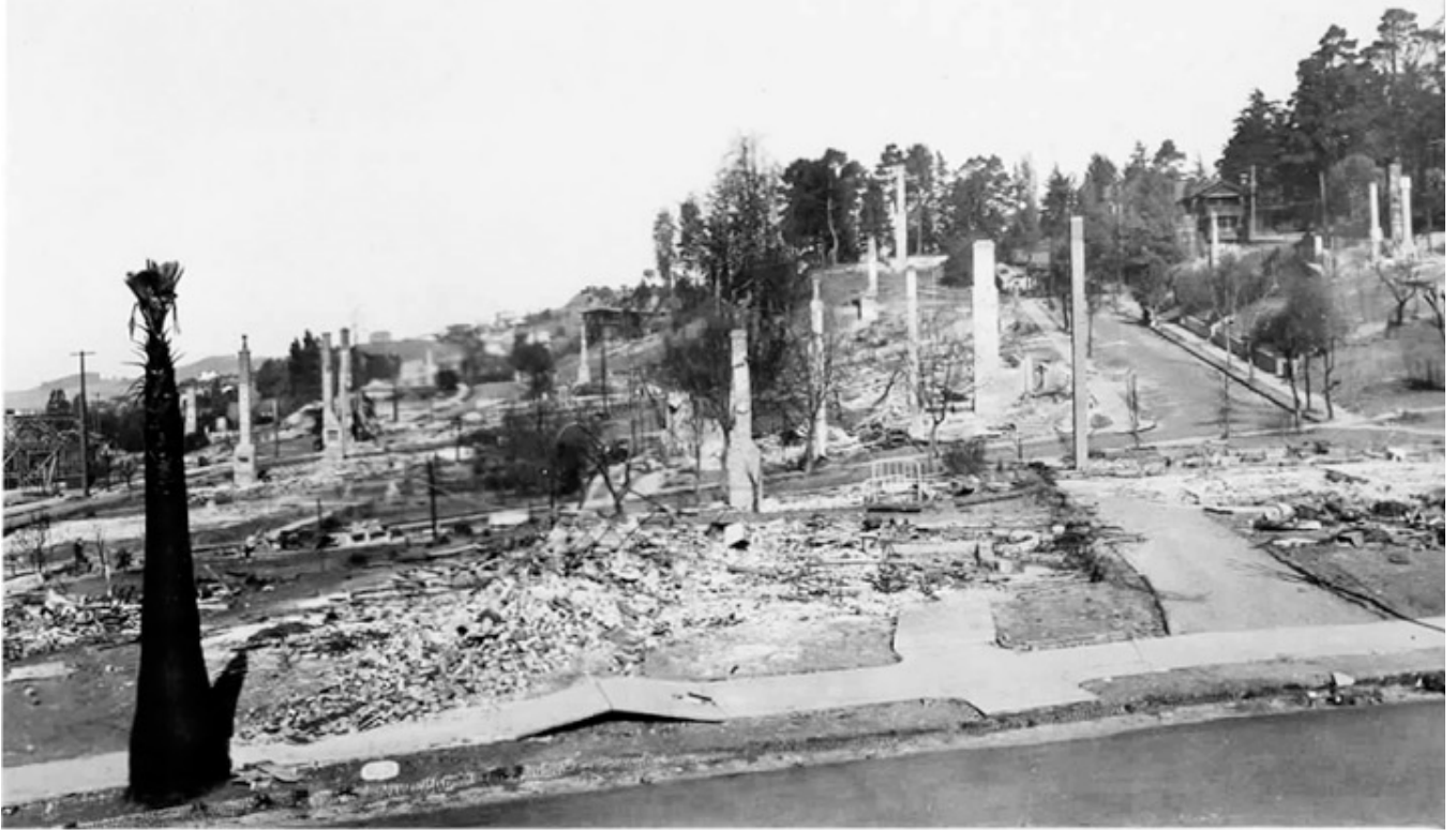
From brick steps of 1562 or 1564 Le Roy Avenue looking north across lots (now the playground of Hillside School) and up Buena Vista Way to the Hyde lot. Sunday, November 4, 1923.
