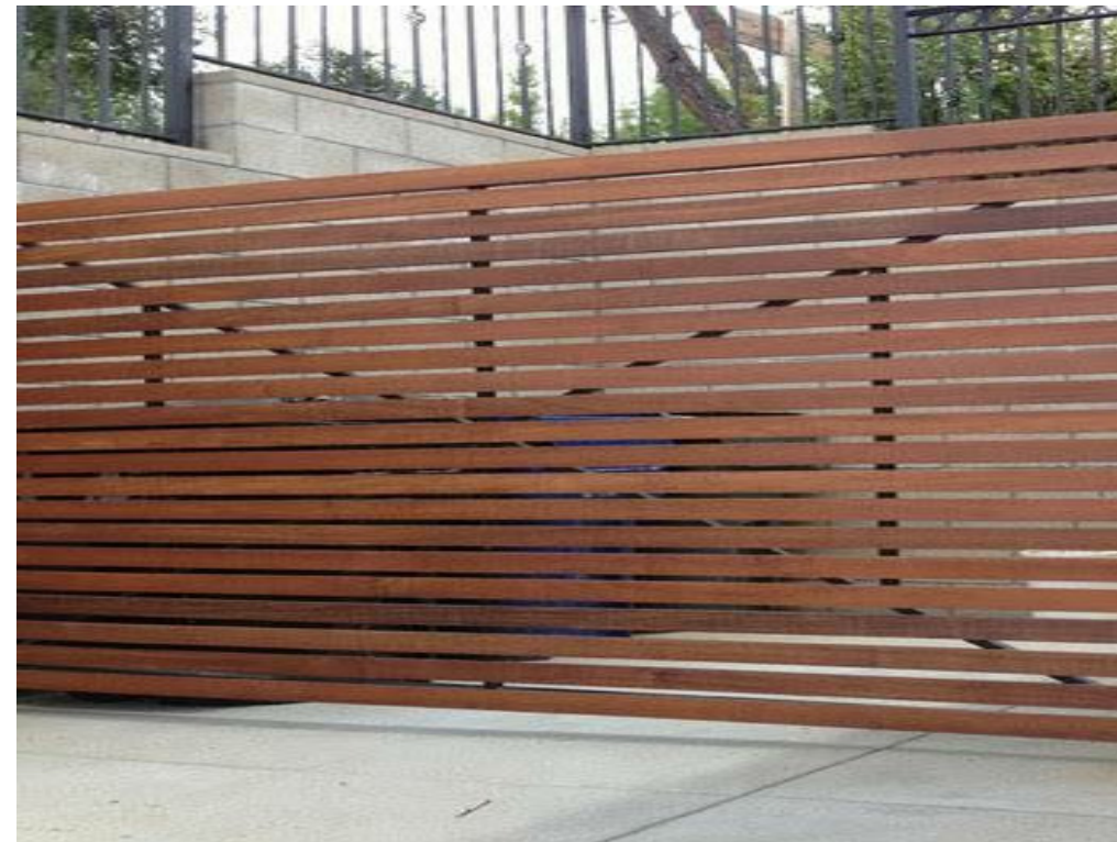
CEDAR FENCE ALONG PROPERTY LINE
