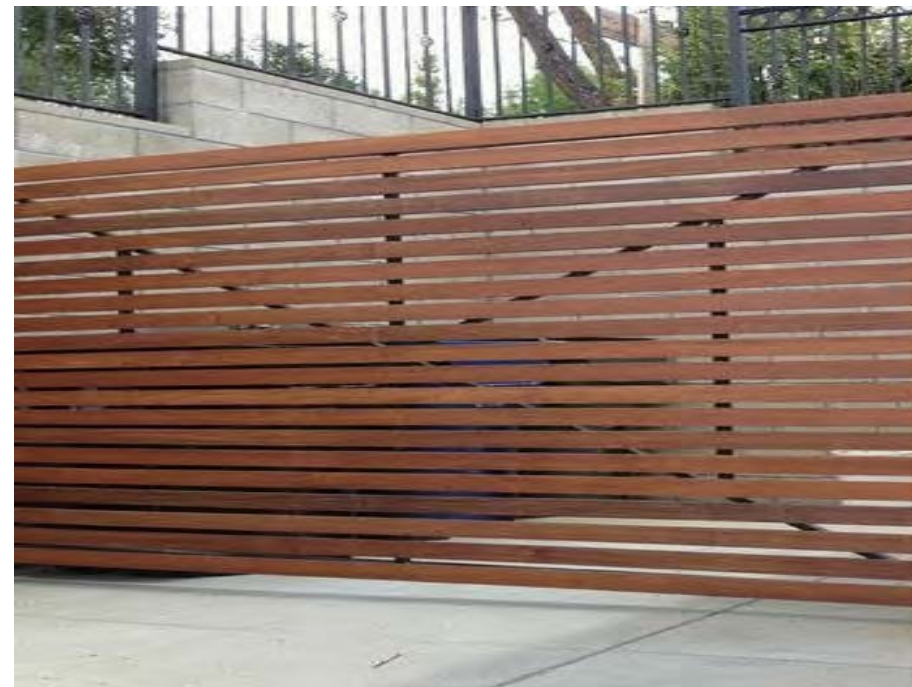
CEDAR FENCE ALONG PROPERTY LINE
