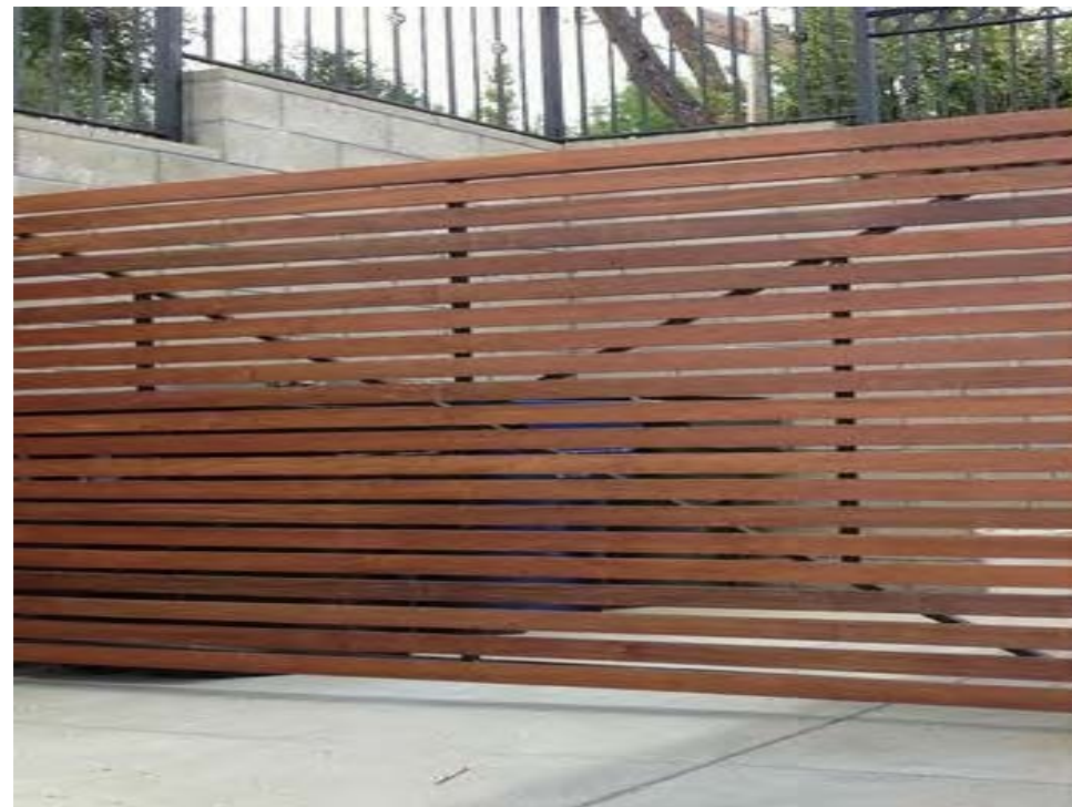
CEDAR FENCE ALONG PROPERTY LINE
