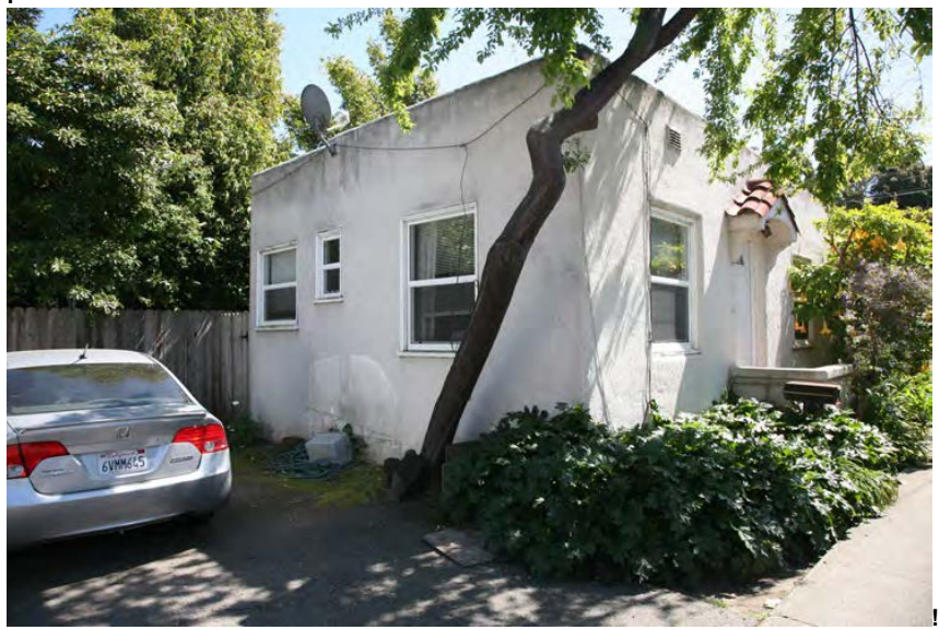
Rear view of 1163 Hearst Avenue, looking southeast (April 2016)
