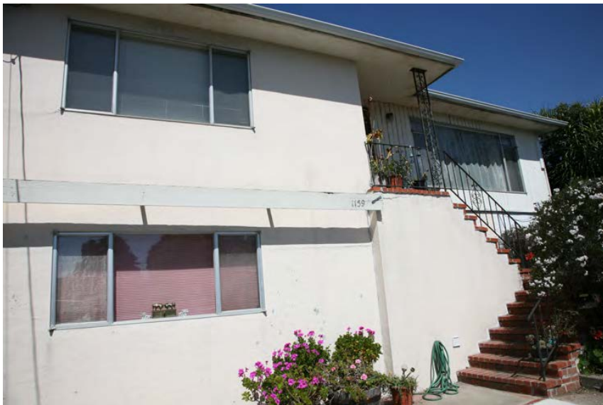
1159 Hearst Avenue, entrance detail, looking northeast (April 2016)
