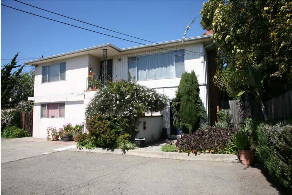
1159 Hearst Avenue, south facade, looking northwest (April 2016)
