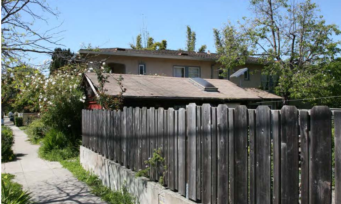
East façade, 1173 Hearst Avenue, looking northeast (April 2016)
