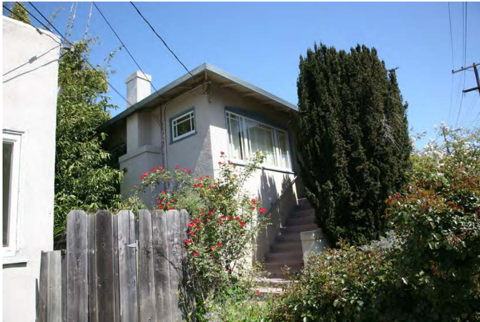
Detail of south and west facades, 1173 Hearst Avenue, looking northeast (April 2016)
