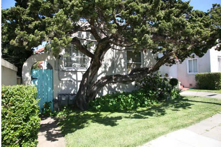
Detail view of 1155 Hearst Avenue, looking northeast (April 2016)
