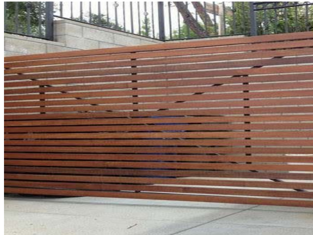
CEDAR FENCE ALONG PROPERTY LINE
