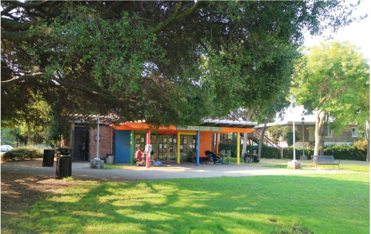
Figure 5 Overview of Willard Park Clubhouse, north perspective
