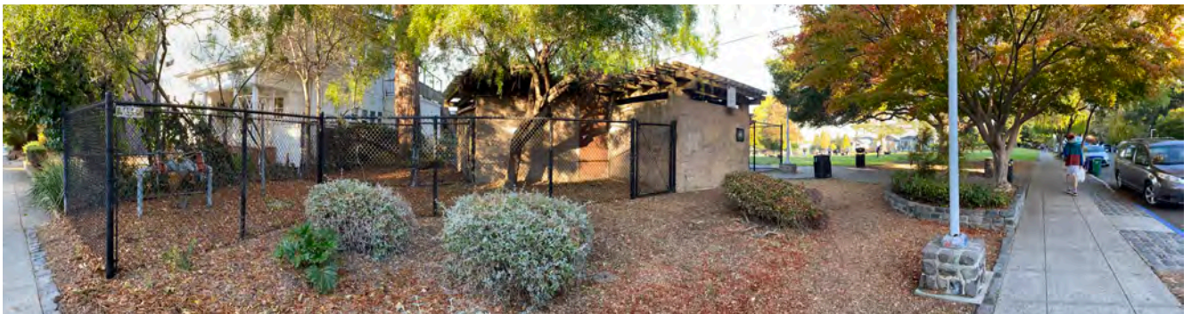
Southeast of proposed clubhouse site - behind existing restroom by Hillegass Ave.
