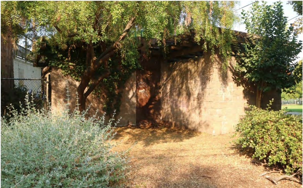
Figure 4 Rear (southeast) elevation of the clubhouse; the concrete block walls house a restroom added to the building in the 1990s
