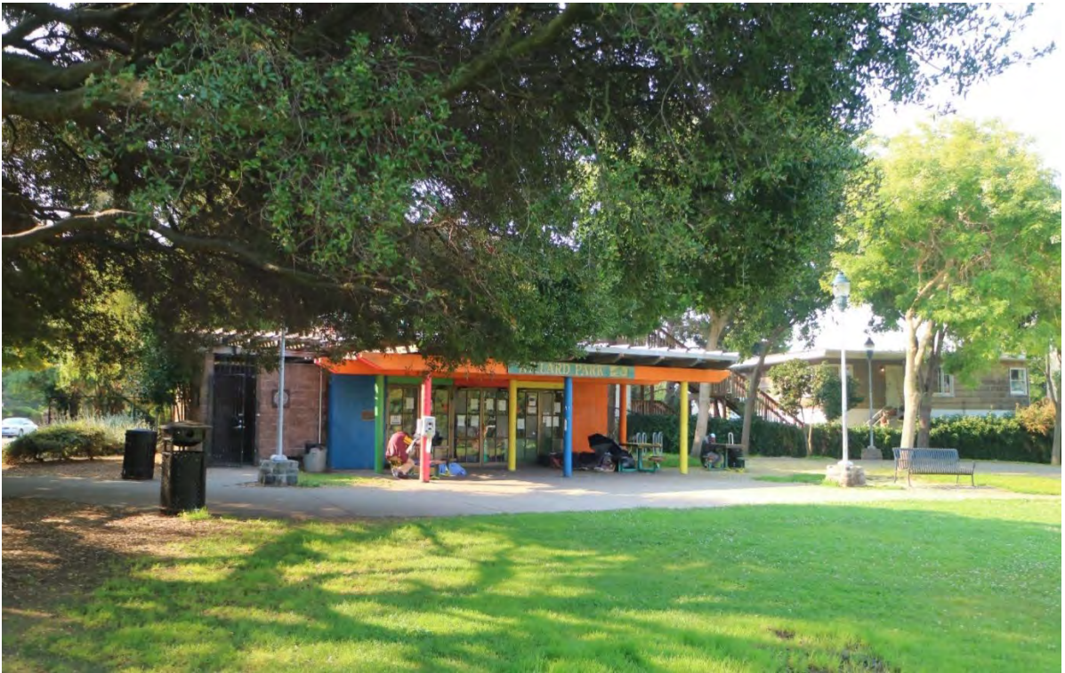
Figure 5 Overview of Willard Park Clubhouse, north perspective
