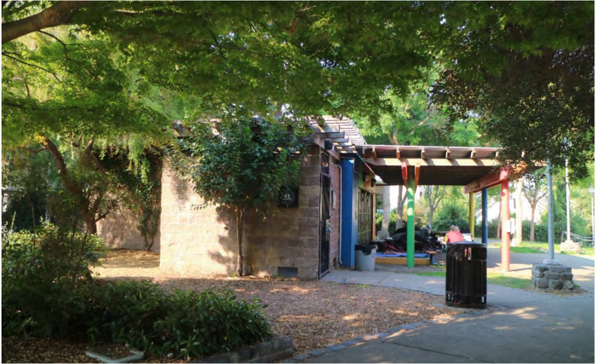
Figure 3 Eastern entrance to park and clubhouse, east perspective
