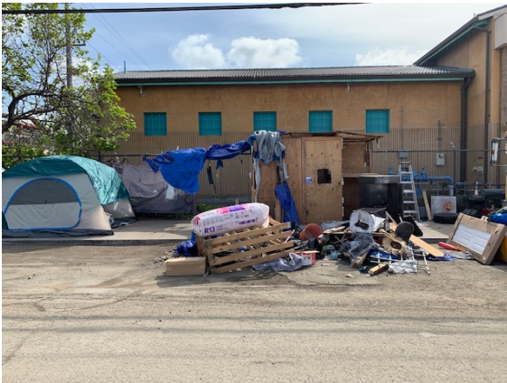
2 nd and Page (Unsafe Structure)- Before
