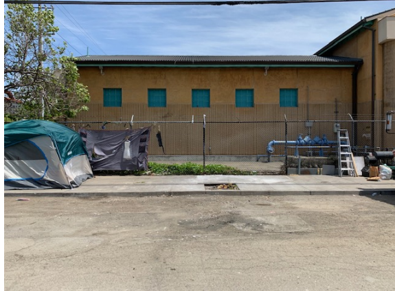
2 nd and Page (Unsafe Structure)- After
