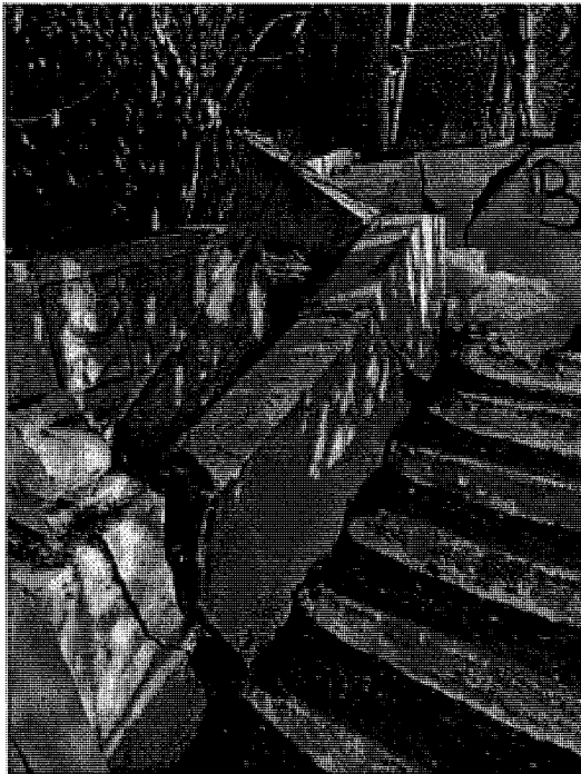
Fig.4 – 639 Arlington Ave. – Entry steps on Arlington
