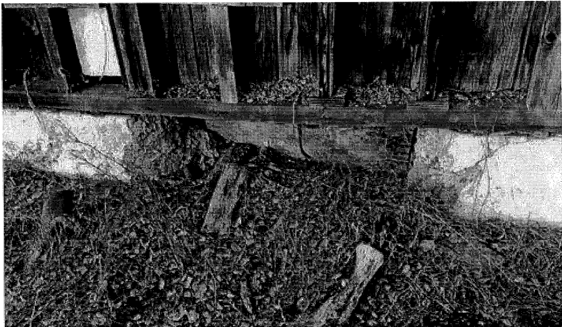
Fig.6 – 639 Arlington Ave. – West side foundations
