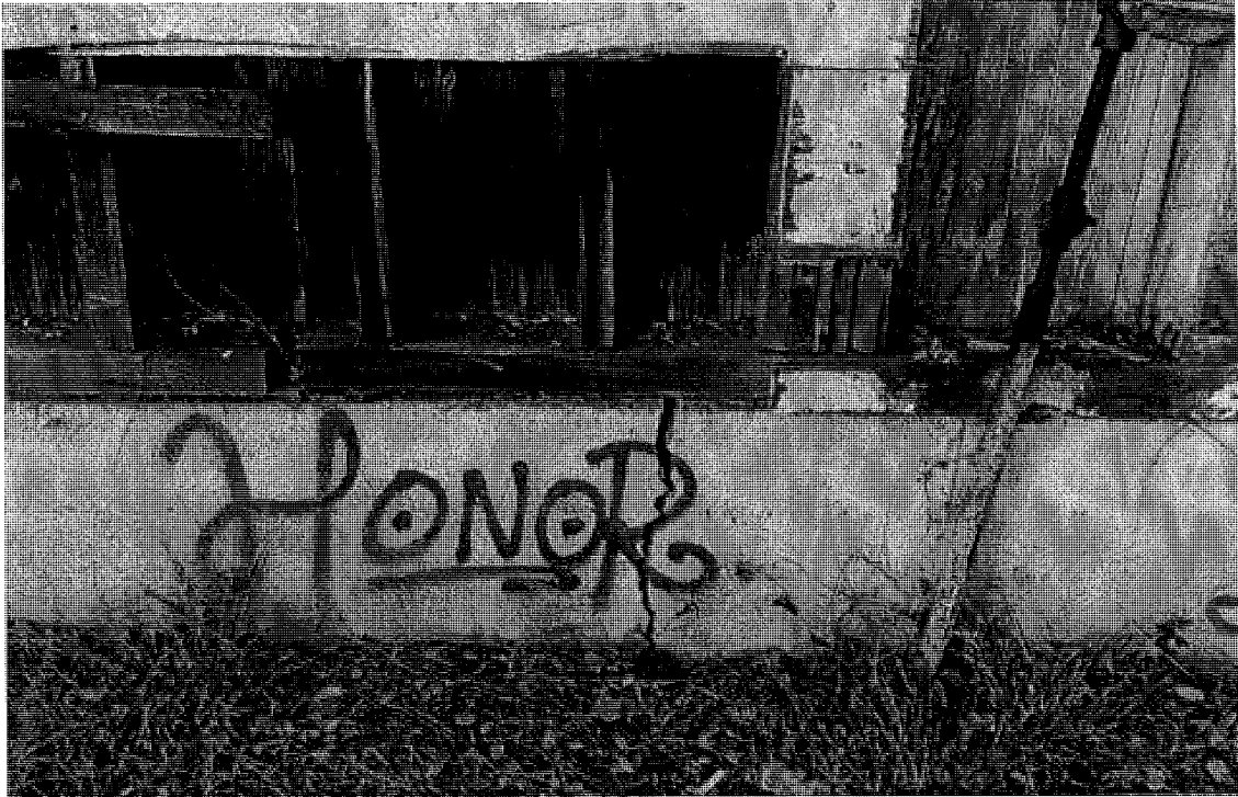
Fig.7 – 639 Arlington Ave. – West side foundations
