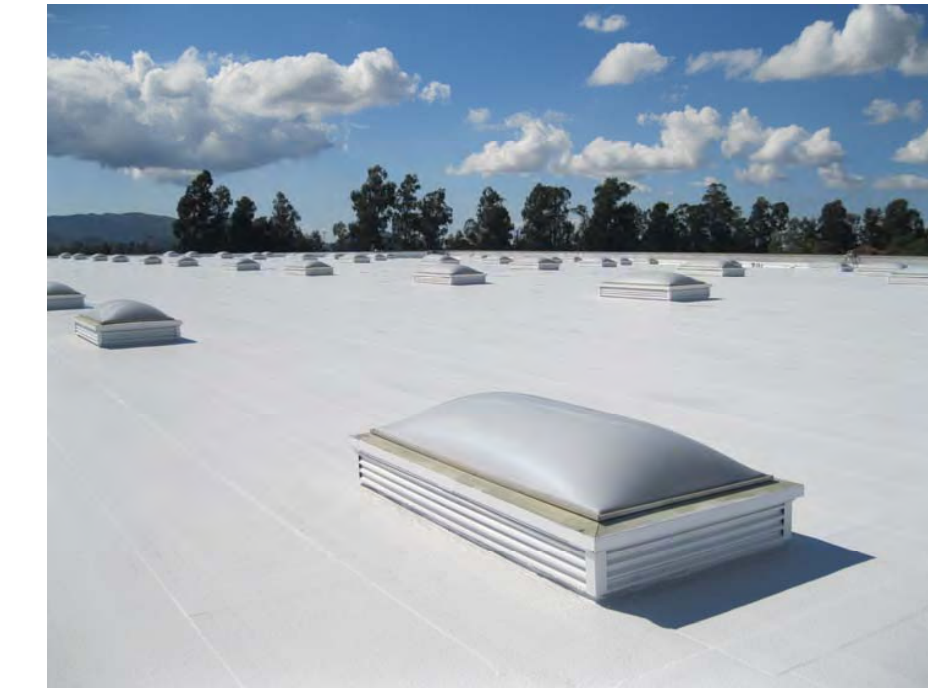
TPO ROOFING - WHITE
