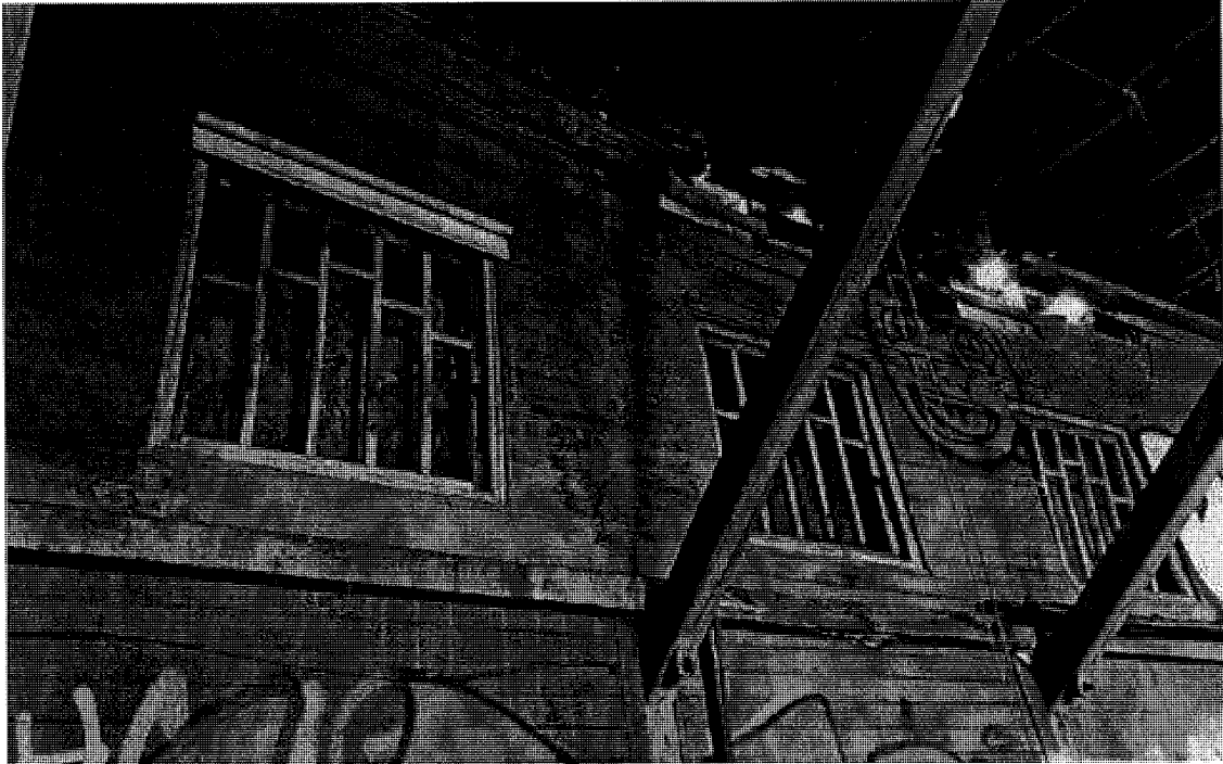
Fig.10 – 639 Arlington Ave. – Interior, east side wall and roof
