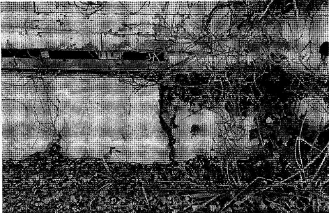
Fig.8 – 639 Arlington Ave. – West side foundations
